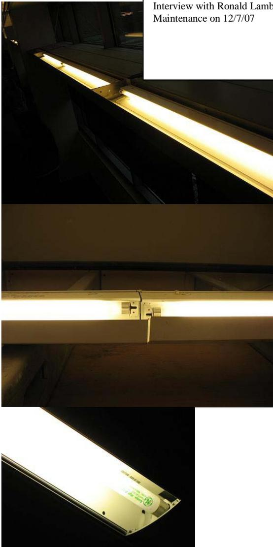
A tool is needed to change the T5 light bulbs. It needs to attach to the bulb and apply enough torque to twist the bulb in order to change the bulb.
